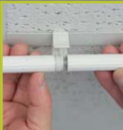
Screw on extensions as desired.
